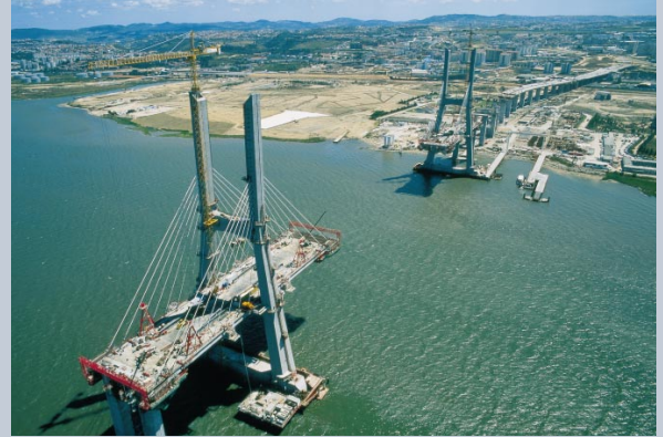
Vasco da Gama Bridge, Portugal
